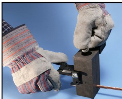
Figure 16. Mold being locked and disk inserted
