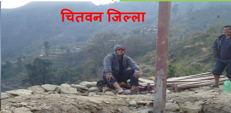
Day 2: Metal Post Erection
