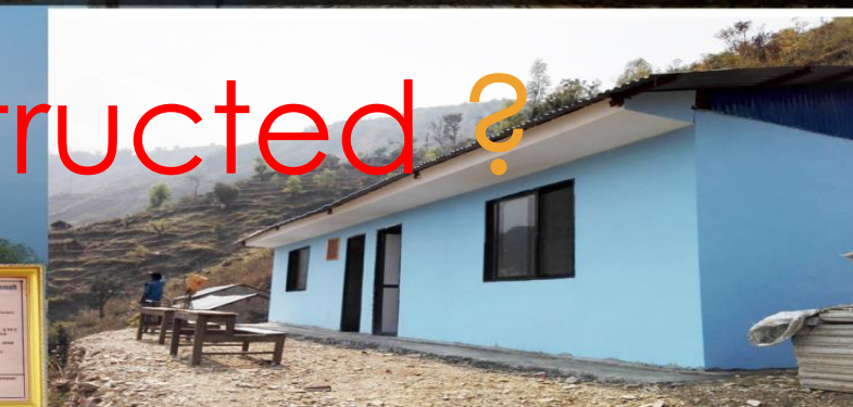
Day 21: Project Completion and Handover
