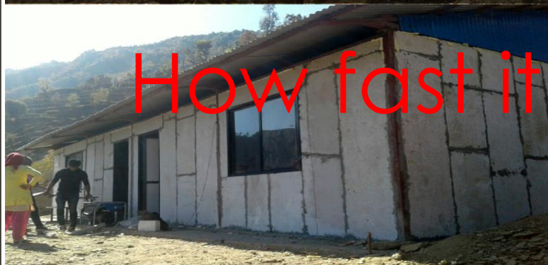
Day 10 & 11: Aluminium Doors & Windows fixation
