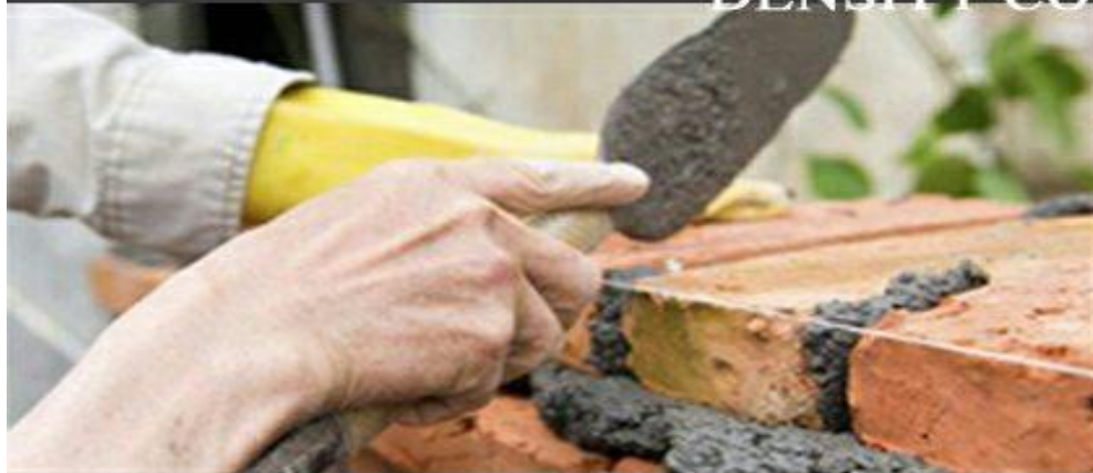
BRICK MASONRY (1900 Kg/m 3 )
