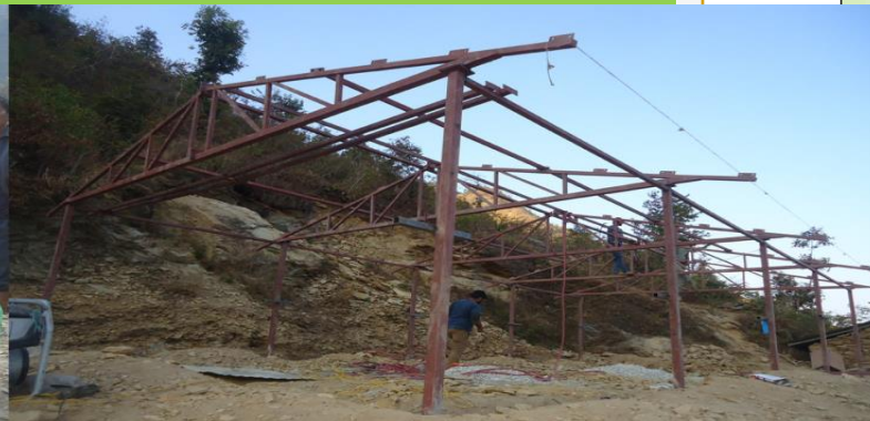
Day 3 and Day 4: Metal Structure & Truss Erection
