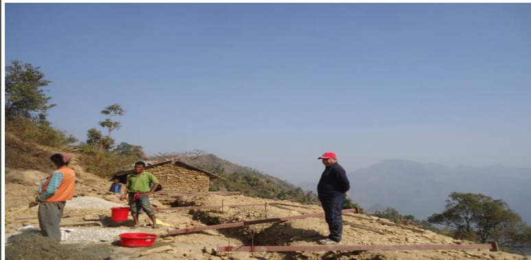
Day 1: Civil Work
