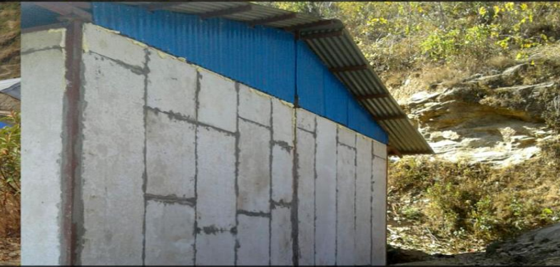
Day 7,8 &9: Gorkha Eco Panel Installation
