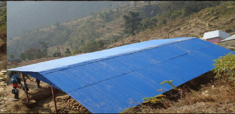
Day 6: Roofing and Truss enclosure
